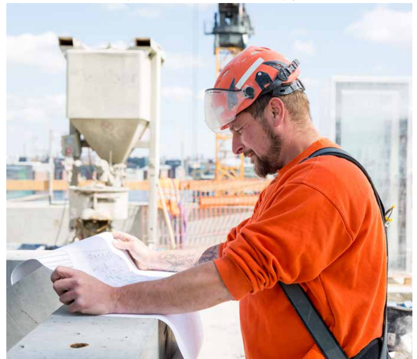
Brian works as a component fitter at PensionDanmark's Sirius construction project and is a member of PensionDanmark
