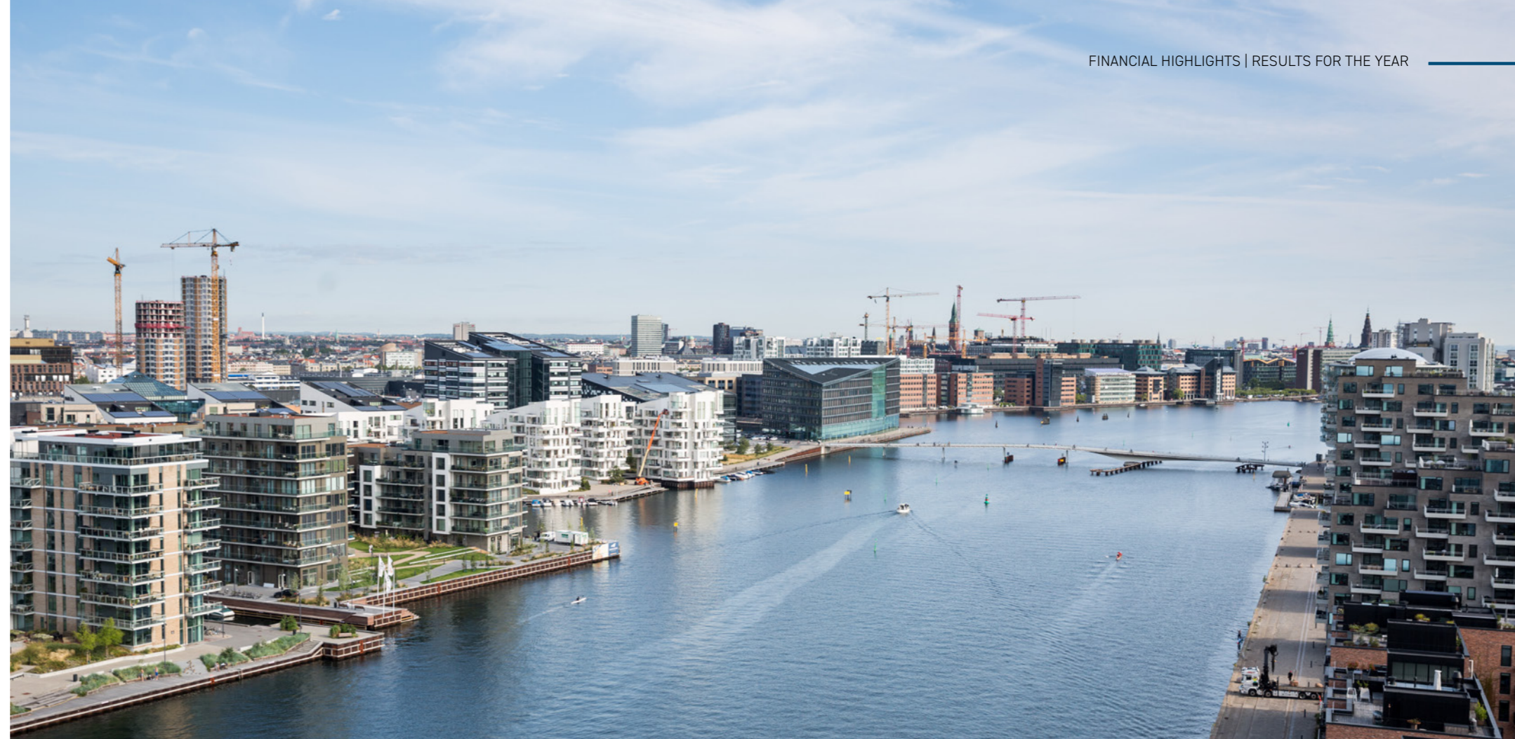
View from PensionDanmark's construction of Sirius in Copenhagen.
