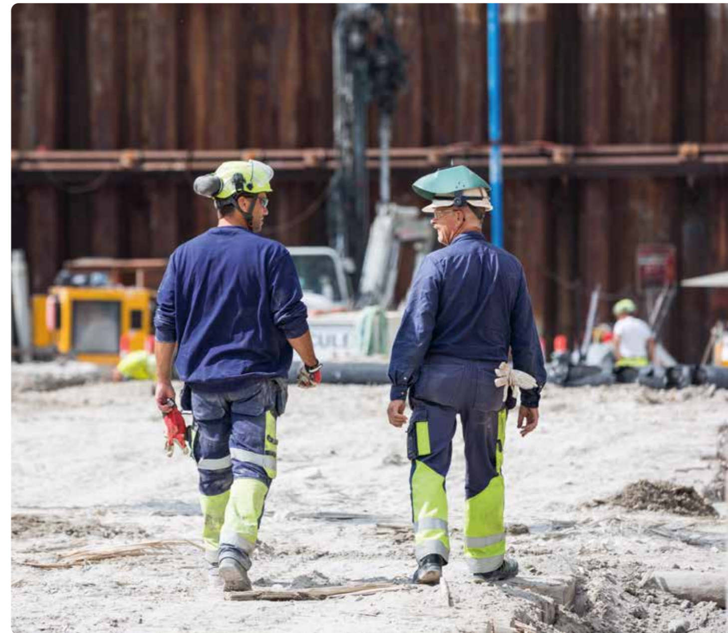
Construction of underground car parks at PensionDanmark's Kronløbsøen construction project
